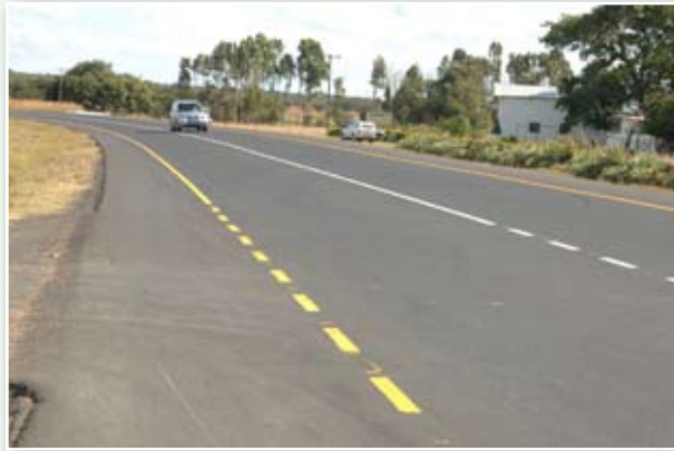
Building of new infrastructure
