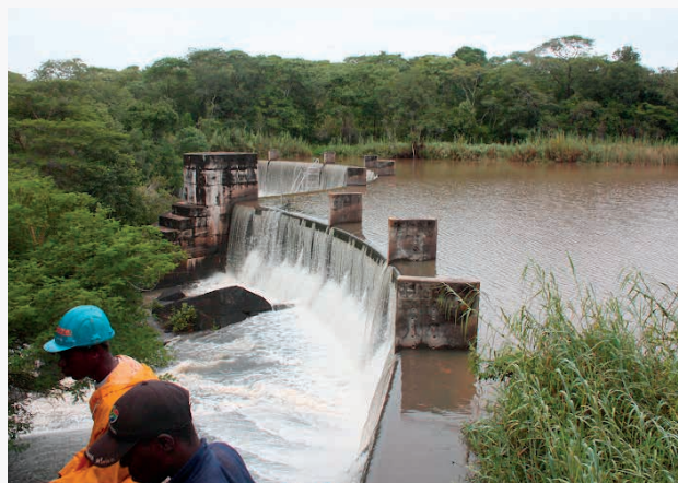
Lunsemfwa Diversion Dam Upgrade
